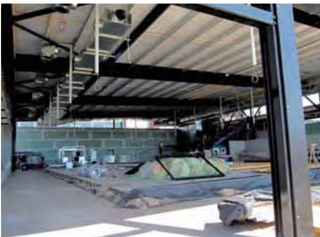
Site visit- Swimming pool enclosure
